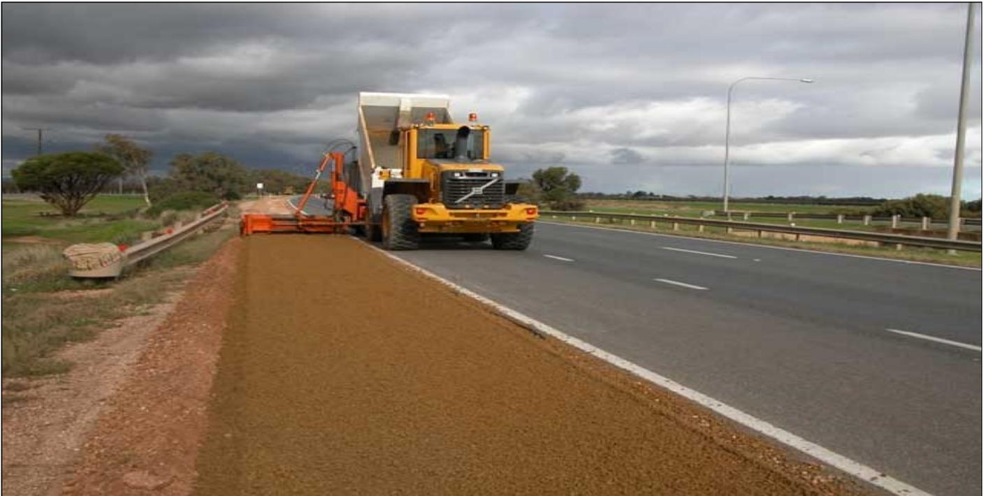
**P.D. Excavations** is equipped with two road wideners, capable of placing material on road shoulders up to 3 metres wide. Automated machine controls are fitted to ensure precise placement of material to exact customer specifications.
